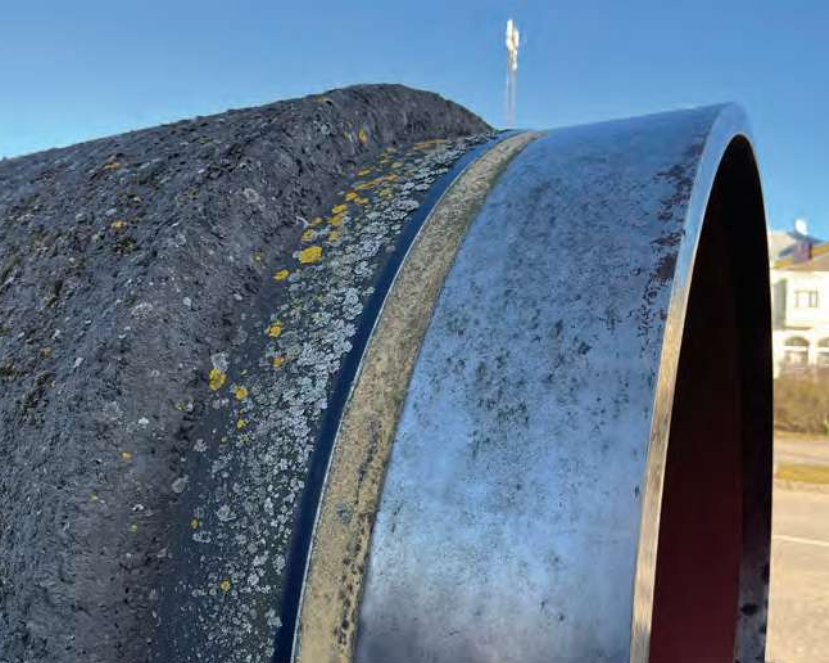
▲ Concrete weightcoating detail of public display of Nord Stream 2 pipeline pipe segment in Hanko, Finland. (April 2025) / CREDIT: B. L. Schmitt
